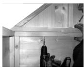
1. Place one gable on top of back panel ensuring the outer edges are flush with shiplap of side panels. Secure from underneath panel framework into gable using 2 x 60 mm screws.
