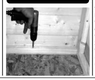
1. Secure wall panels to the floor on the inside of the building using 2 x 60 mm screws for back and side panels and 1 x 60 mm screw for wing panel, preferably into floor bearer.
