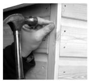
1. Secure remaining three cover strips in position where the panels meet using 3 x 40 mm nails per strip.
