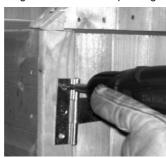
5. Place door into aperture, check door is square and even all the way round and secure in place using 3 x 25 mm screws per hinge.
