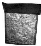
2. Place other roof panel onto the remaining piece of felt, allowing an overhang of approx. 45 mm on three sides and an approx. overhang of 200 mm on the forth side. Fold felt over onto roof panel, except for the side with the approx. 200 mm overhang, and secure in place using felt nails.
