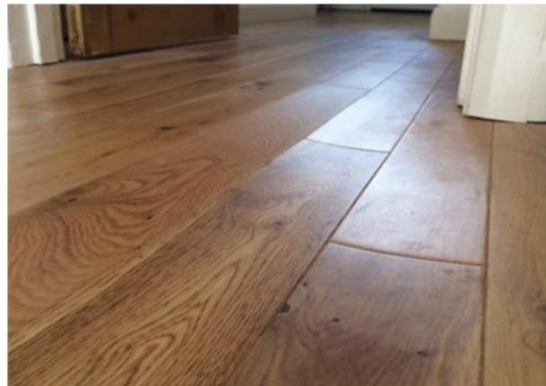
Sometimes the edges of wood flooring boards appear to be rising up to form a ridge between each board. This is known as cupping and is invariably caused by the moisture level below the floor being higher than the top surface. The underside therefore expands more than the top surface causing the edges to push upwards.
