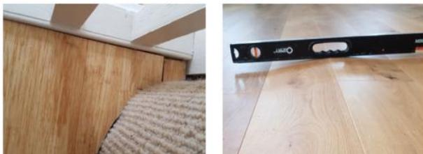
The direct reverse of shrinkage, wood flooring expands as its moisture content increases. Correct expansion gaps around the perimeter will absorb any normal changes, but where exceptional expansion takes place and there is no further room around the perimeter, the floor will sometimes start to push upwards over an area (bridging), or as a pair of boards (tenting).
