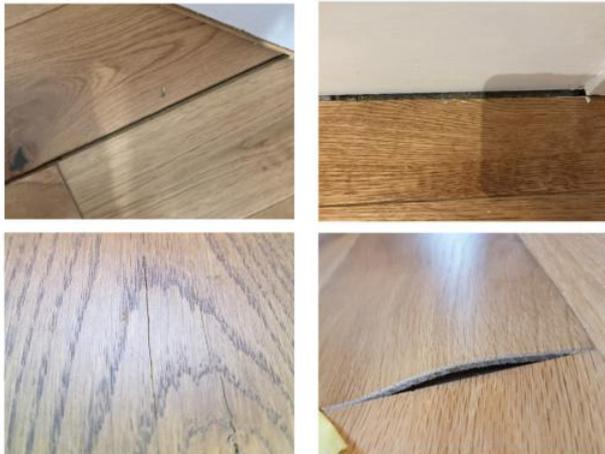
Wood flooring is a hygroscopic material, meaning it will expand or contract according to its moisture content. Where significant shrinkage, gapping, or splitting appears, this is due to a corresponding reduction in moisture level in the flooring. Here are some reasons why this might happen.
