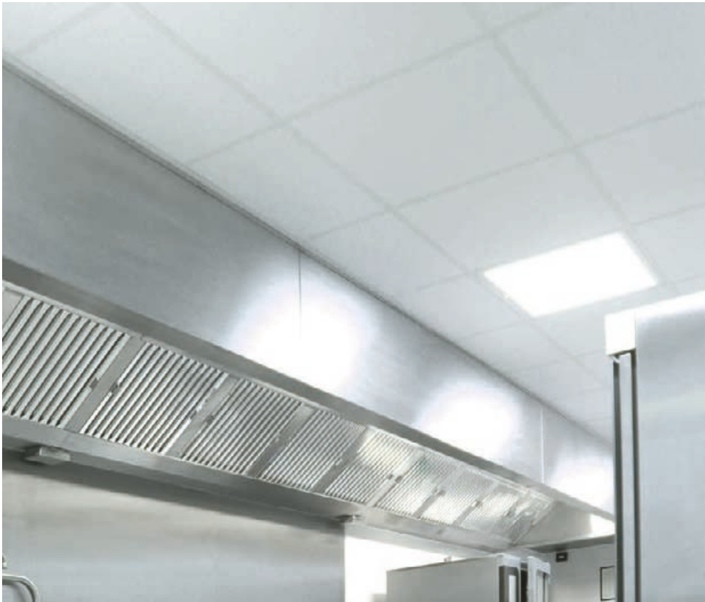
Bristol Hospital UK
