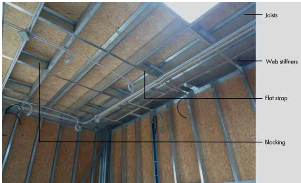
Fig. 5.14: Floor: Indication of joists and web stiffeners
