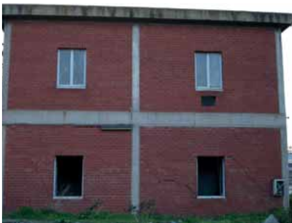
Fig. 4.6: Masonry infill walls in a reinforced concrete frame
