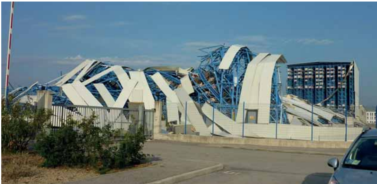
Fig. 4.35: Property loss risk: Damage to scaffolds in storehouses, 2012 Emilia Earthquake, Sant'Agostino, Italy /Marco Savoia/
