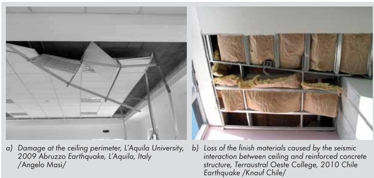
Fig. 4.32: Damage to suspended lightweight steel gypsum board ceilings
