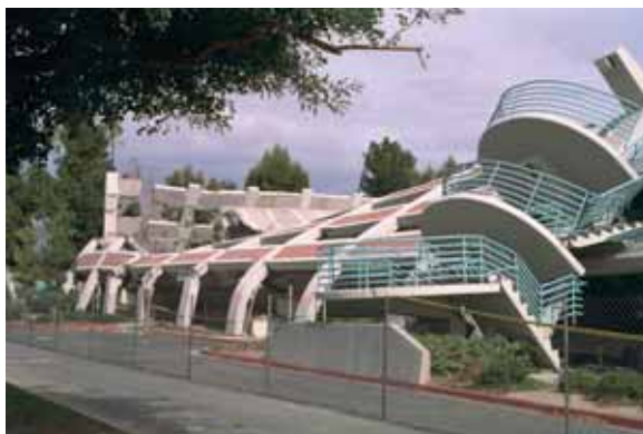
Fig. 2.4: 1994 Northridge earthquake /Department of the interior/U.S. Geological Survey/
