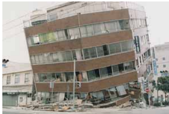
Fig. 2.5: 1995 Kobe earthquake /Kobe City/
