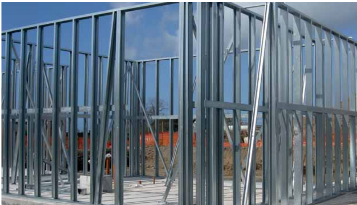
Fig. 5.3: Typical steel framing
