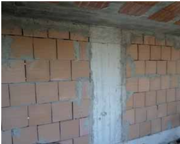
Fig. 4.10: Interior heavy partition wall
