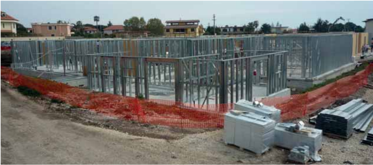
Fig. 5.57: CFS frame construction of stick-built structures
