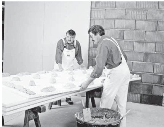
Fig. 3.4: Application of a composite board /Knauf Gips KG/
