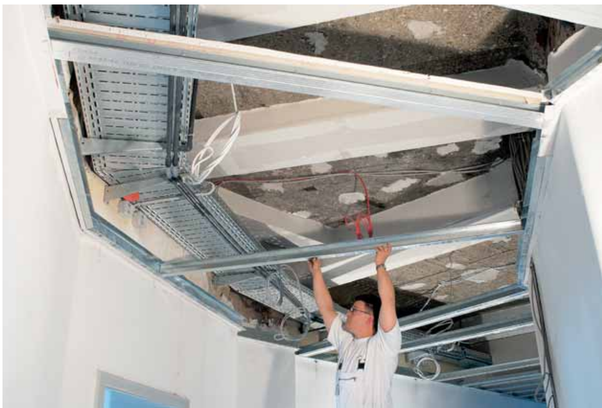
Fig. 3.14: Installation of a free-spanning suspended ceiling /Knauf Gips KG/
