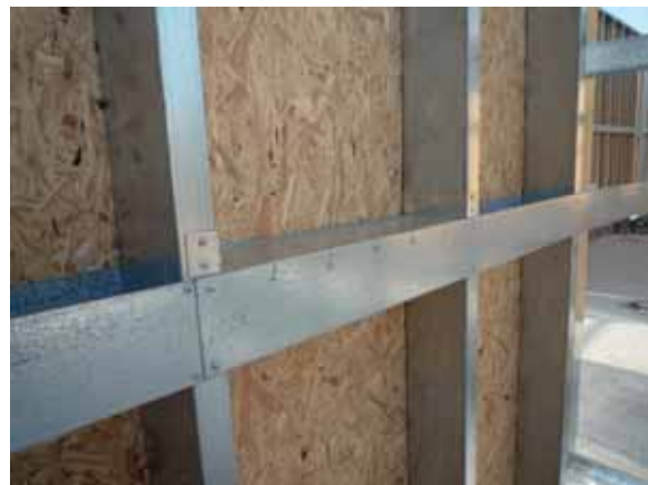
Fig. 5.16: Wall lateral restraint
