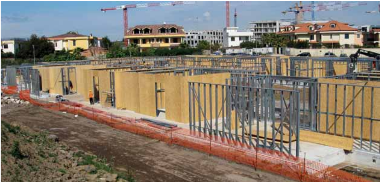
Fig. 5.58: Cladding boards fixing
