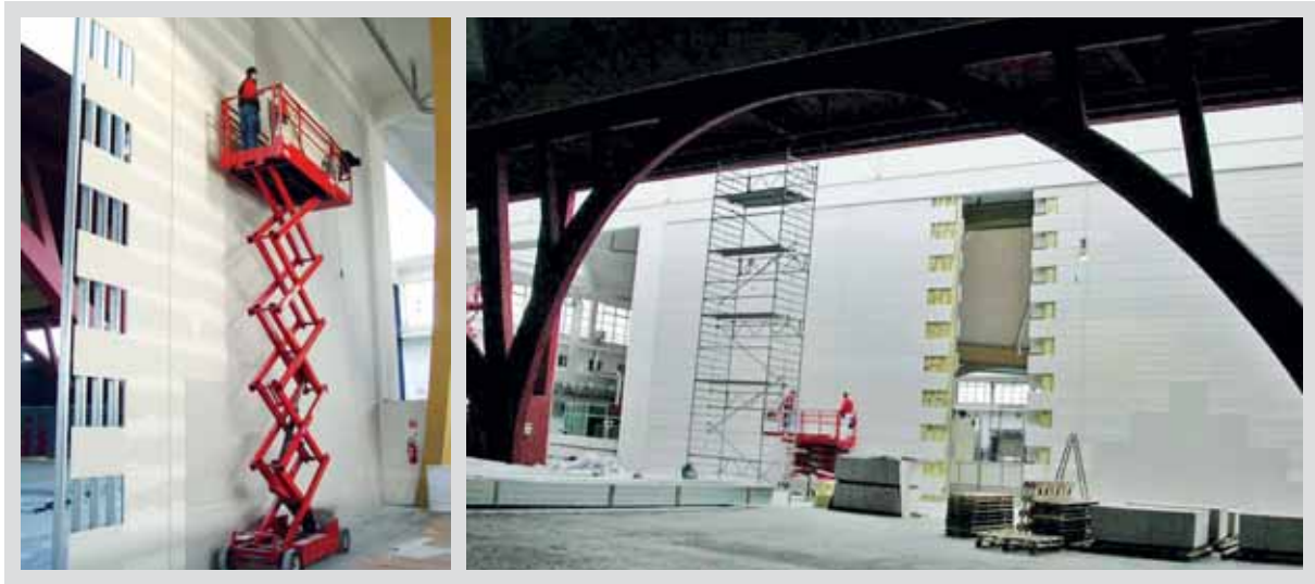
Fig. 3.6: Installation of an 11 m high stud partition /Knauf Gips KG/
