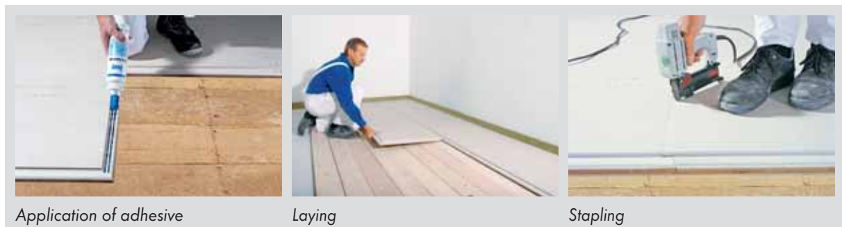
Fig. 3.16: Laying of pre-fab floor screed /Knauf Gips KG/
