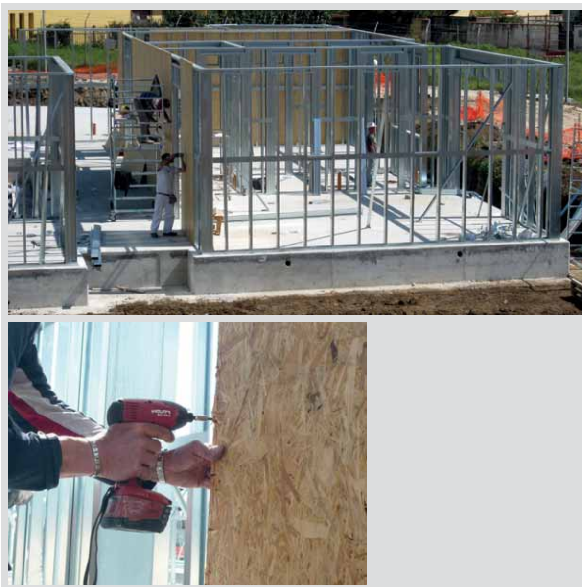
Fig. 5.13: Cladding system and cladding-to-frame connection
