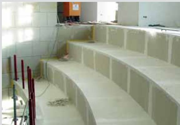
Fire protection with Fireboard during construction
