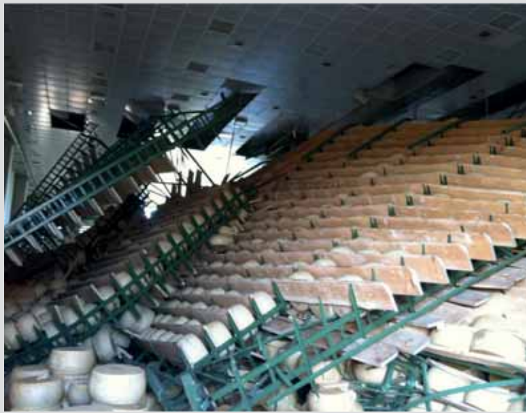
a) Overturning of shelvings in a cheese storehouse, 2012 Emilia Earthquake, Mantova, Italy /Marco Savoia/
