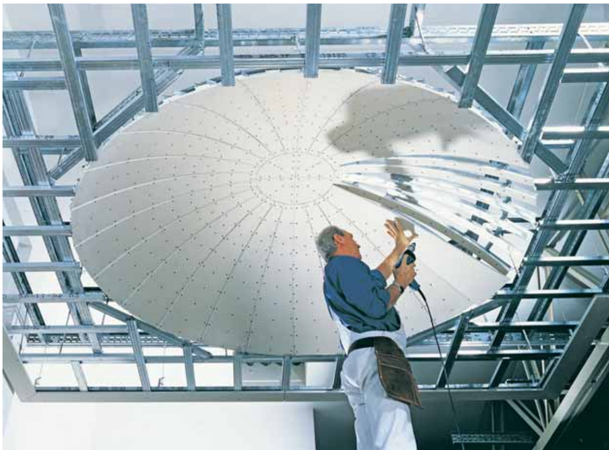
Fig. 3.13: Installation of a suspended ceiling with integrated cupola /Knauf Gips KG/
