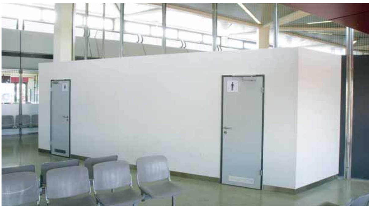
Fig. 3.21: Sanitary cell in the airport Berlin - Tegel /Knauf Gips KG/
