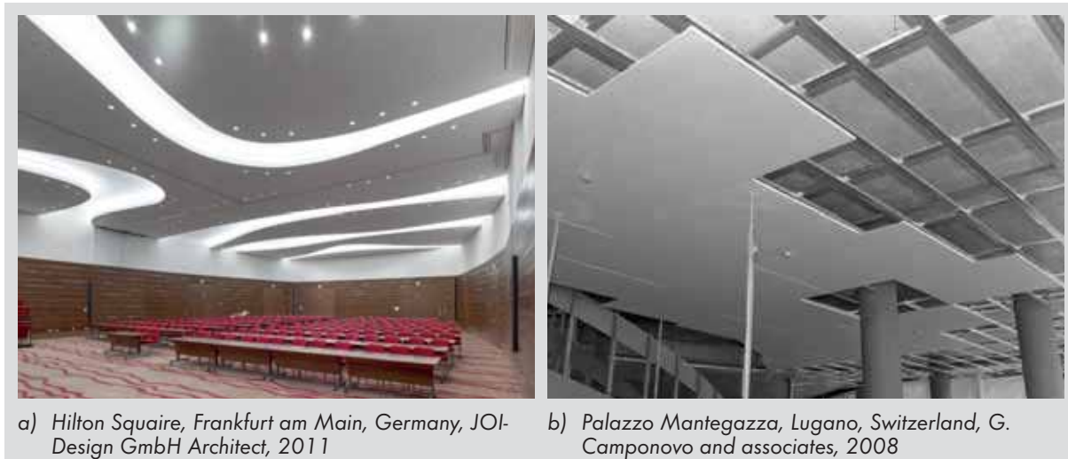
Fig. 4.14: Suspended lightweight steel gypsum board ceilings
