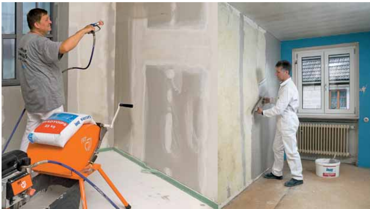
Fig. 3.33: Machine application and smoothing of Readygips /Knauf Gips KG/
