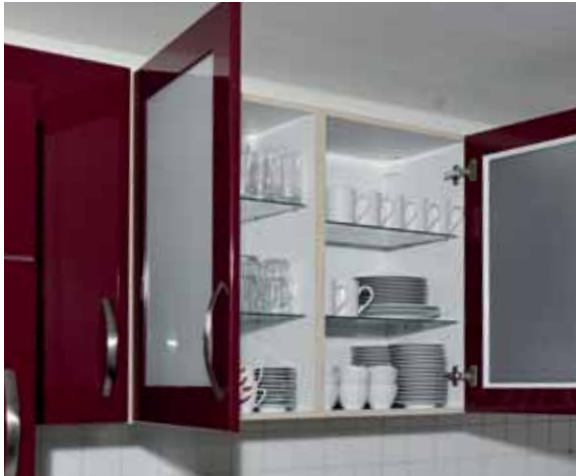
Fig. 4.15: Cabinet with asymmetric centre of load gravity to the surface of the drywall partition /Cambodunum Film GmbH/
