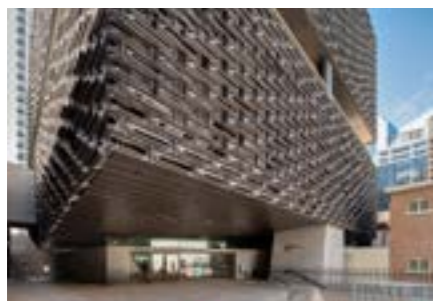
Tai Kwun Centre | Hong Kong, China
