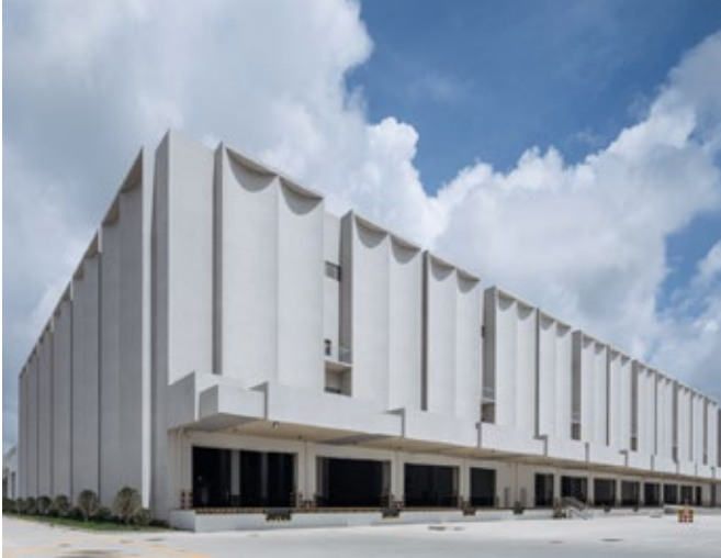
Lingang Warehouse | Shanghai, China
