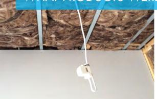
Earthwool® ceiling batts, R5.0 were installed in the ceilings; this R-Value is higher than the recommended minimum standard for ceilings and will provide high thermal performance as well as contribute towards the 6 star energy rating.
