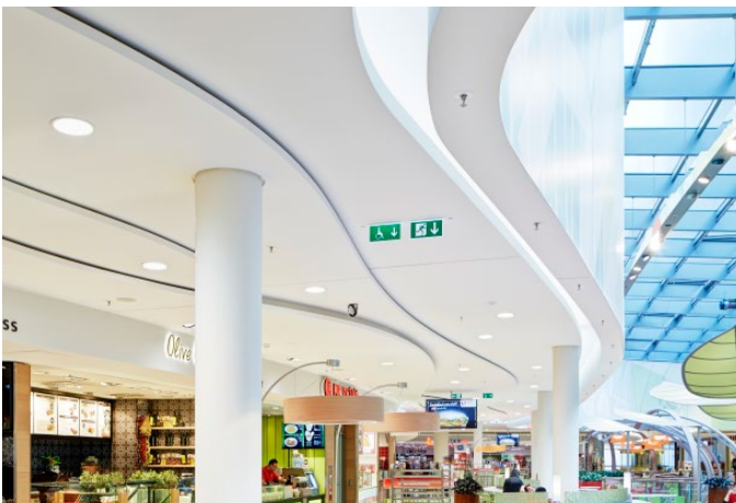
Staggered ceiling levels break up the large surfaces. The prerequisite for a perfect surface was created by Knauf Horizonboards with tapered edges around the perimeter.
