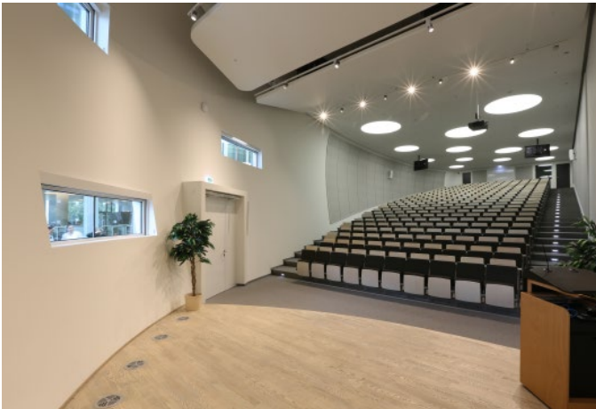
A look into the Auditorium Maximum with interior plastering work to quality level Q4. (Photo: Knauf/Halama)
