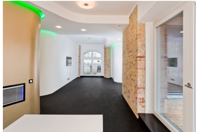
The party walls on the basis of the Knauf system W115.de as dual stud partitions, clad with Knauf Diamant and Knauf Piano, achieve a weighted sound reduction index R'_w of 65 dB. This is 12 dB more than the minimum requirement according to DIN 4109.
