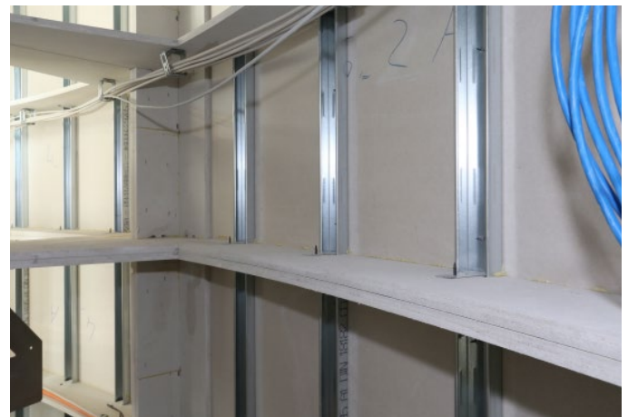
With millimetre precision: Connection point of two modules beside one another and two modules above one another.
