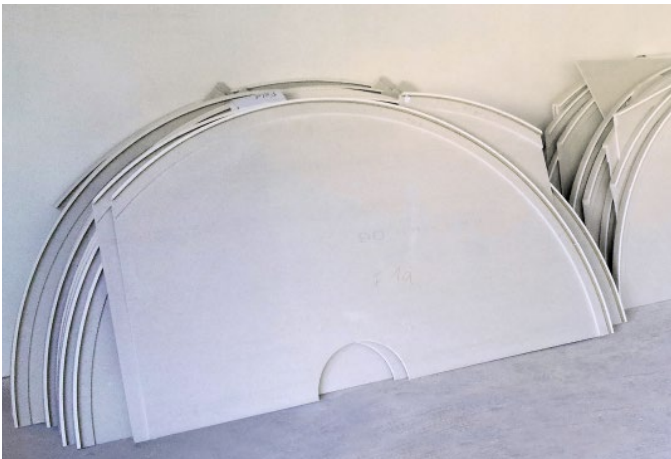
Preassembled kit for complete prefabricated canopy (Photo: Jaeger Ausbau)
