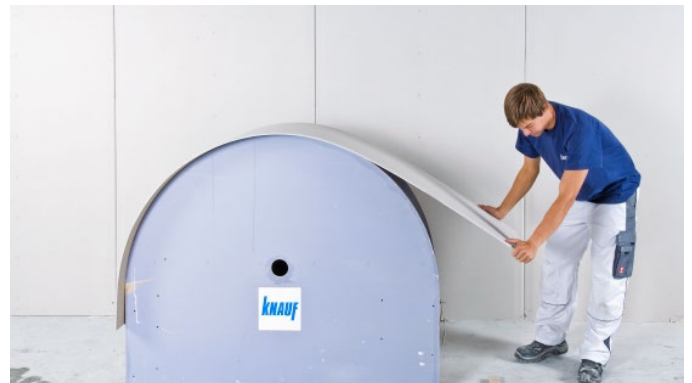
Image 4: Fix board on template
