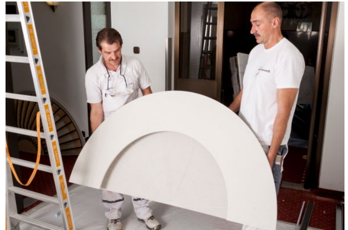
The individual elements of the dome were supplied in segments.
