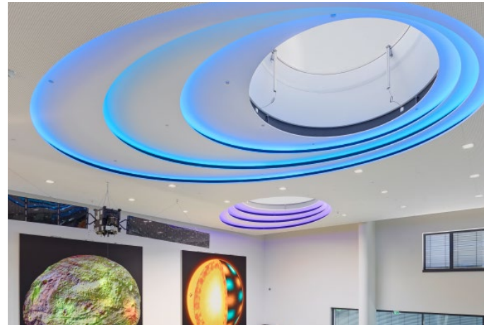
A sophisticated ceiling construction characterizes the foyer of the Max-Planck-Institute for Solar System Research in Göttingen. (Photo: Knauf/Braun)
