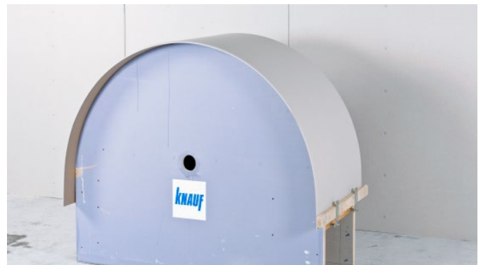
Image 4: Fix board on template
