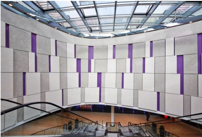
The coloured curved elements of the relief structures on the wall surfaces curved at varying radii making up the mall eyes consist of prefabricated gypsum boards.
