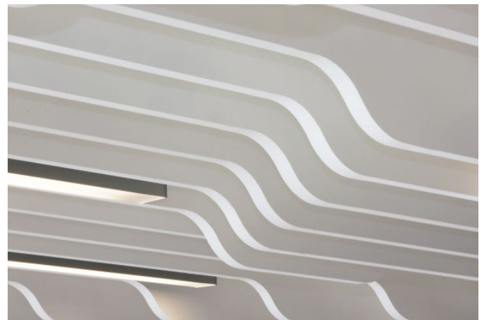
Perfect wave fronts on the ceiling of the large auditorium in the InnovationsCampus of the HK Hamburg.
