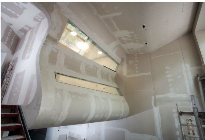
Drywalling from the lower to mezzanine floors. (Photo: Gallandi)
