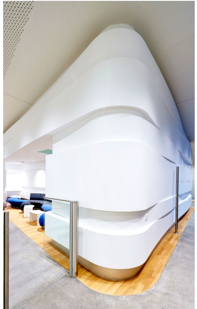
Like an aircraft nose, the drywall construction made of Knauf design units projects into the lounge of the ZAL Finkenwerder.
