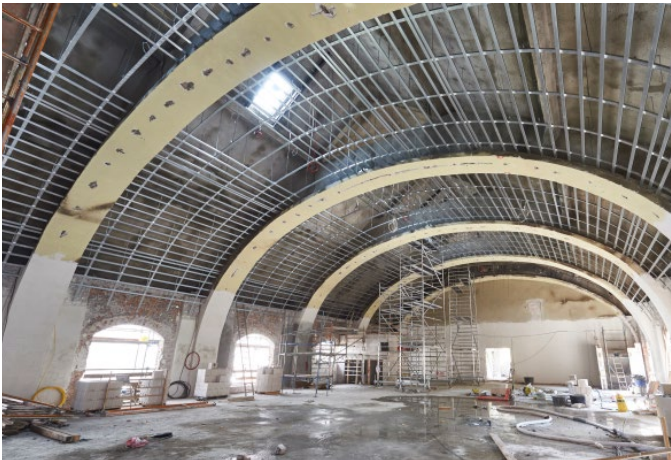
The grid onto which the perforated boards of the Knauf Acoustic Board Ceilings are screw fixed is adapted to fit between the beams.
