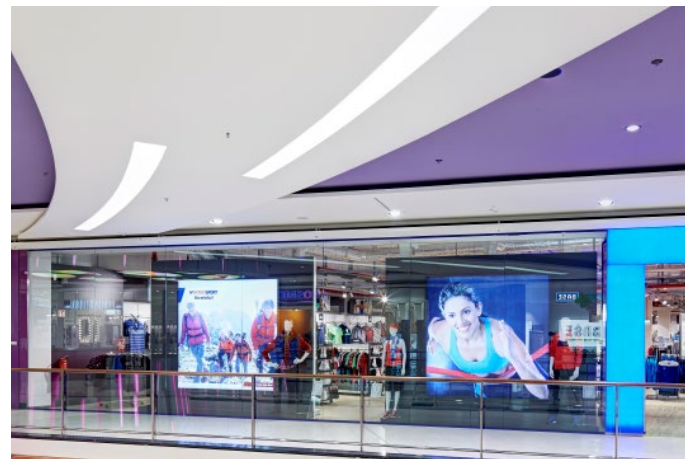
Free formed ceiling rafts with integrated curving recessed lighting put the passageways above the galleries into the right lighting perspective. Ten to twelve individual elements were required to construct the ceiling raft.
