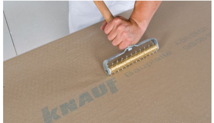
Image 2: Place board on template
