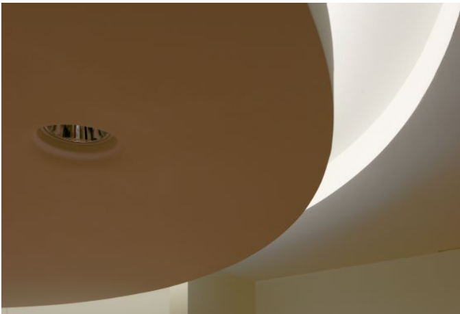
Curved to perfection. This ceiling landscape was made possible by prefabricated design units.
