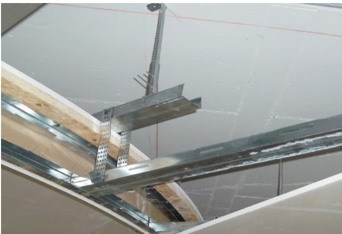
Detail split level ceiling (Photo: Ruben Peter Ausbau GmbH)
