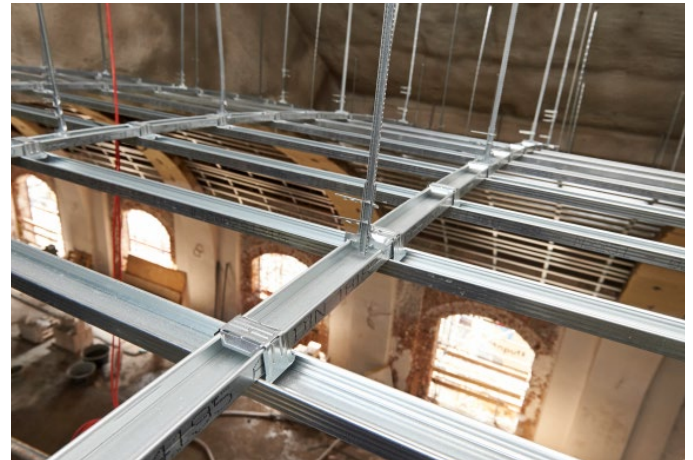
The curved carrying channels of the grid were prefabricated in the factory to the required radii and delivered as an exact fit.
