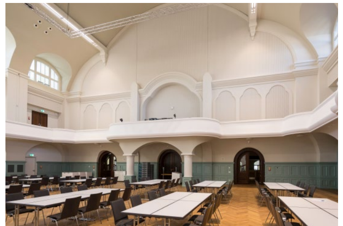
The rear of the large hall is a sound absorption surface and implemented using drywall.
