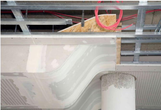
Split level ceiling in S arch form
