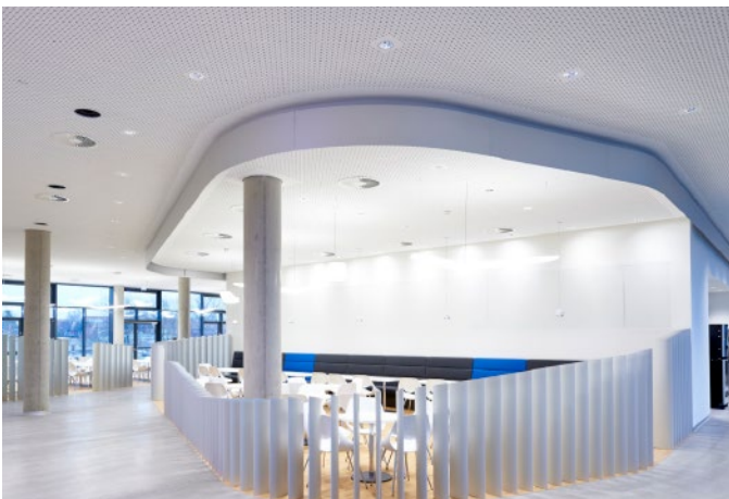
Rounded Knauf design units are also located on the ceiling of the canteen areas in the reception area of ZAL, sectioned off by aluminium pedestals.
