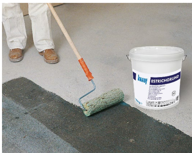
Figure 82: Application of Estrichgrund screed primer
