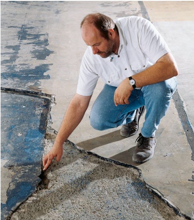
Figure 105: Check the substrate
