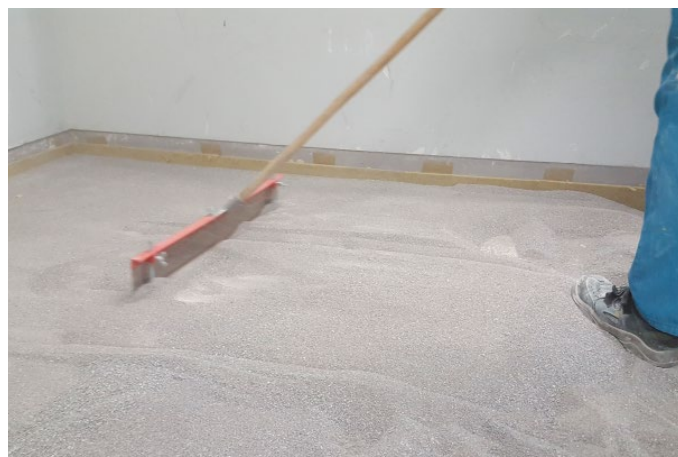
Figure 38: Installation of Schwere Schüttung heavy-duty acoustic infill
