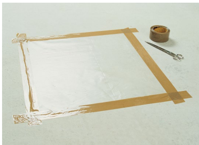
Figure 69: Initial inspection of drying with foil on the heating floor screed
