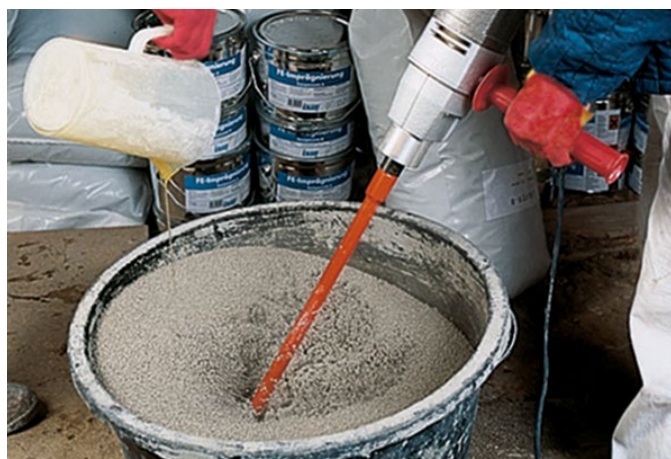
Figure 37: Mixing in the tub is quick and does not require any great effort.
