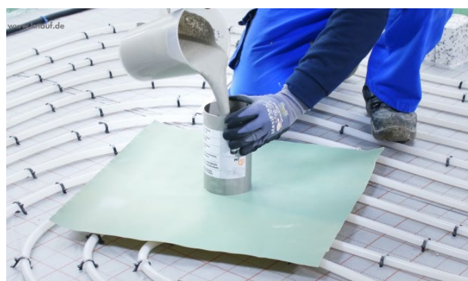
Figure 54: Fill the consistence checking tin with mortar
