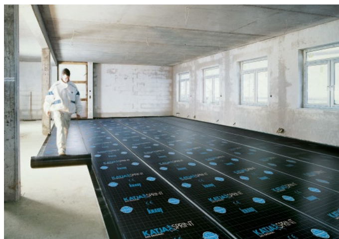
Figure 31: Katja Sprint Abdichtungsbahn sealing membrane: Quick to lay with a high yield
