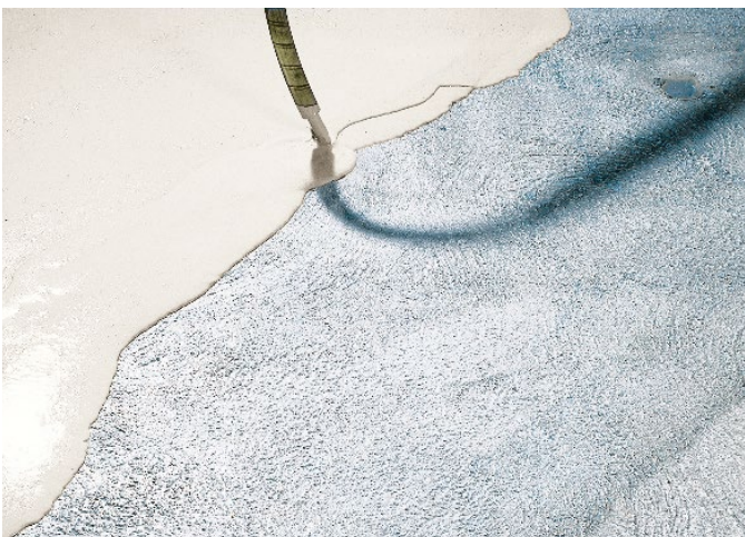
Figure 84: Machine application of N 410
