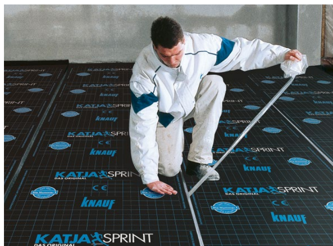
Figure 32: Sealing the long joints by removing the protective film
