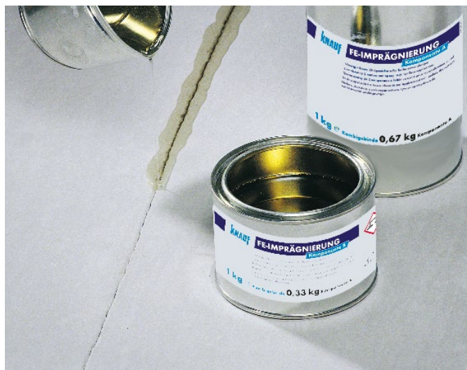
Figure 81: Filling cracks with epoxy resin
