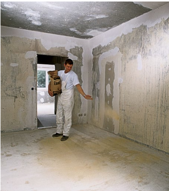
Figure 106: e.g. Bonding layer interspersed with silica sand
