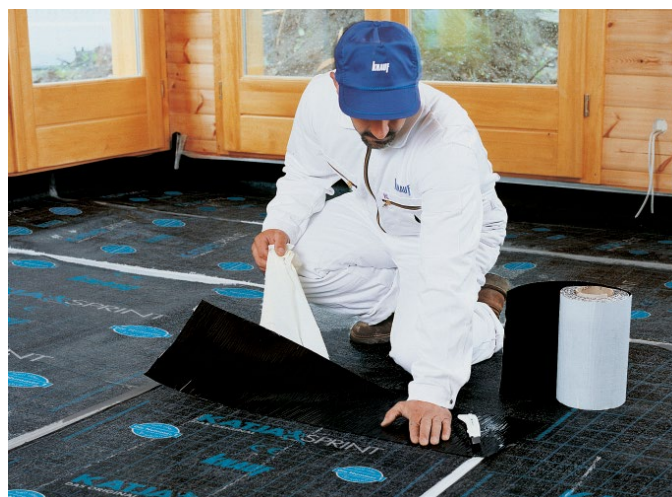
Figure 33: Sealing of front end joints with Katja Sprint connector tape
