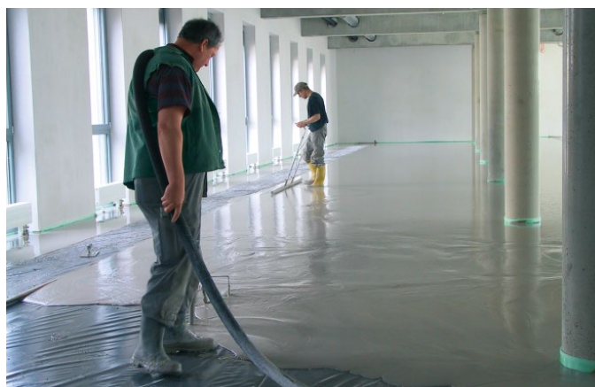
Figure 24: Installation of flowing screed on the prepared raised access floor construction
