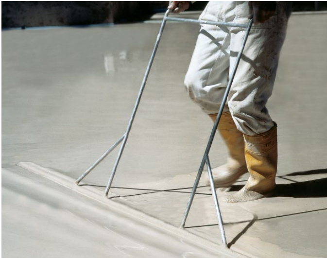
Figure 59: Working with a dappling bar
