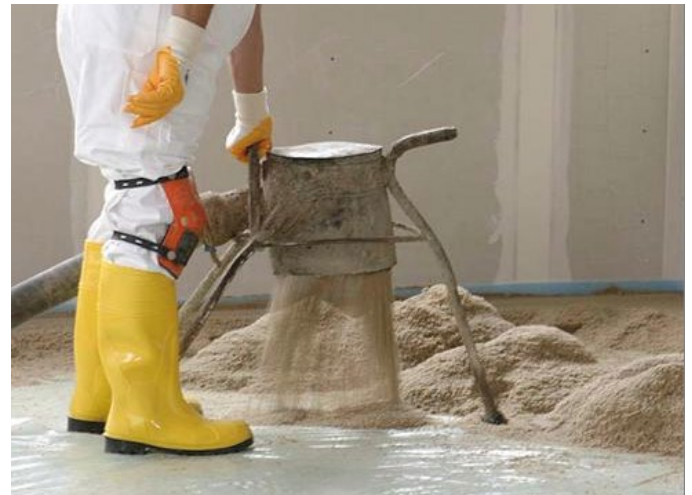
Figure 93: Application with a compressed air conveyor
