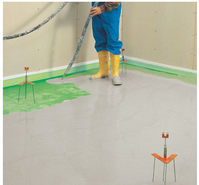
Figure 58: Pouring the screed
