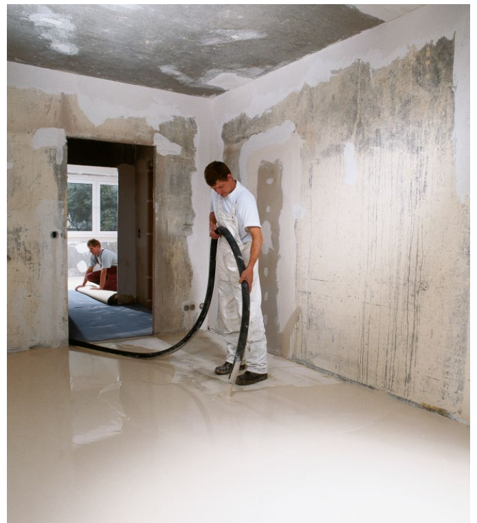
Figure 108: e.g. Machine application of N 440
