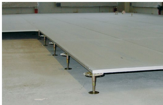
Figure 23: Installation of pedestals and sheathing units
