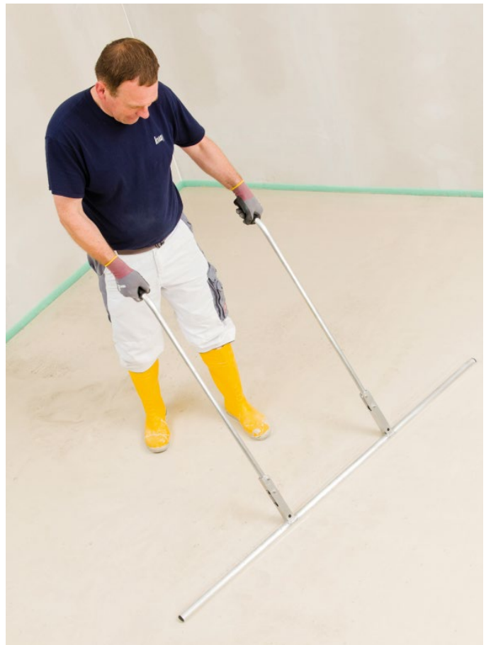
Figure 100: Dappling the screed
