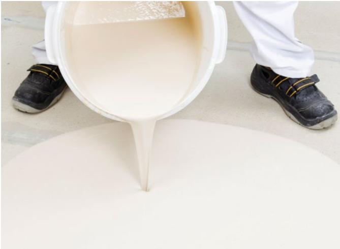
Figure 83: Manual application of N 410
