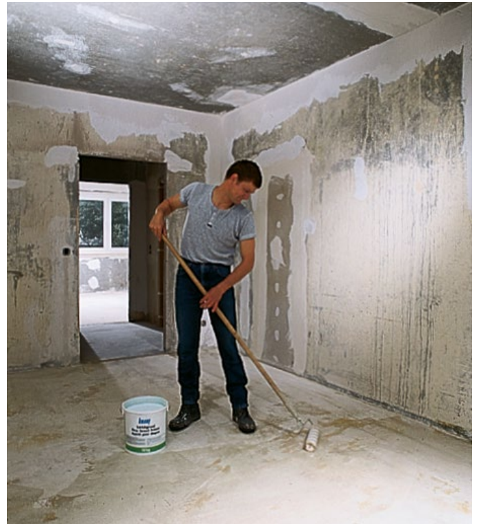
Figure 107: e.g. Prime with Estrichgrund screed primer
