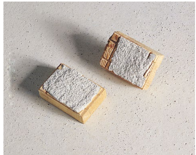
Figure 80: Parquet and screed failure patterns
