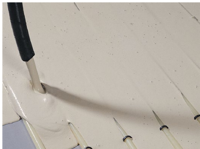
Figure 19: Apply the heated screed
