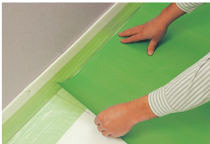
Figure 17: Laying Knauf Schrenzlage synthetic coated kraft paper
