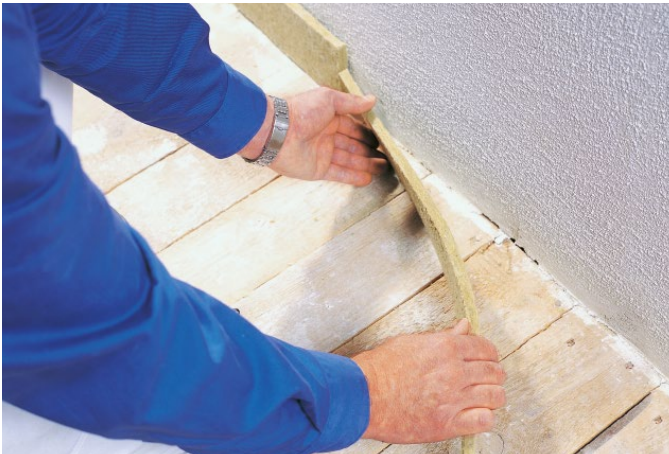
Figure 40: Application of mineral wool edge insulation strips with fire protection requirements
