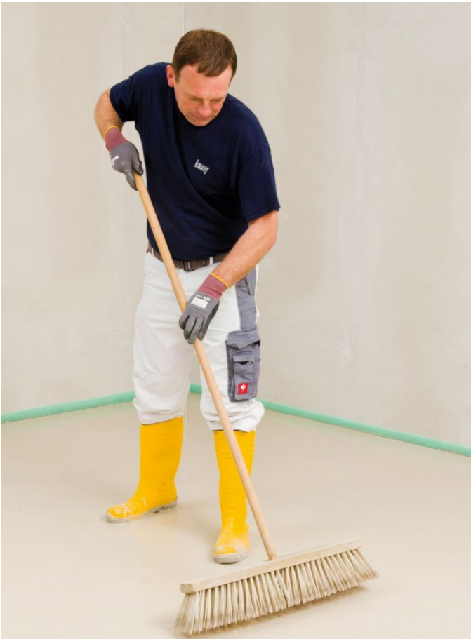
Figure 101: Working with a screed brush
