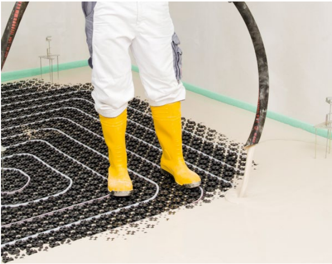
Figure 99: Pouring the N 440 mortar
