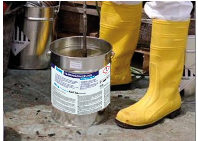
Figure 92: Mixing of the epoxy resin with a mixer
