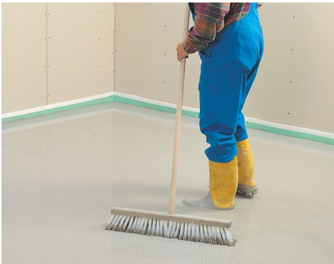
Figure 60: Working with a screed broom
