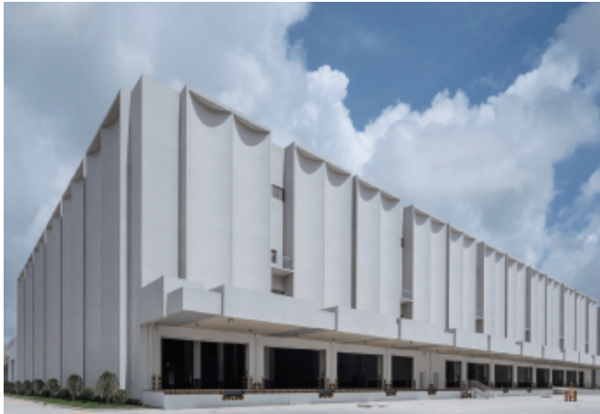
Lingang Warehouse Shanghai, China
