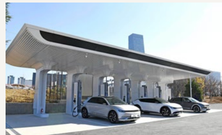
E-pit charging station
